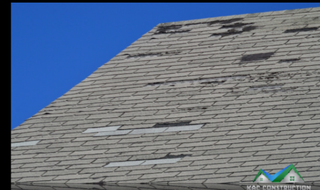
Missing Shingles
