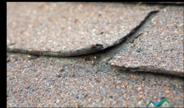
Shingles Buckling
